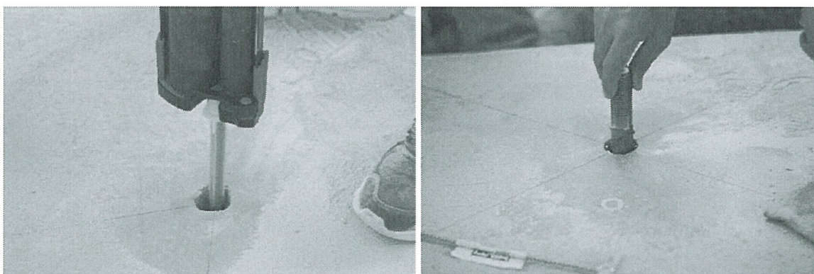
Figure 2: Adhesive Anchors (RE100)
